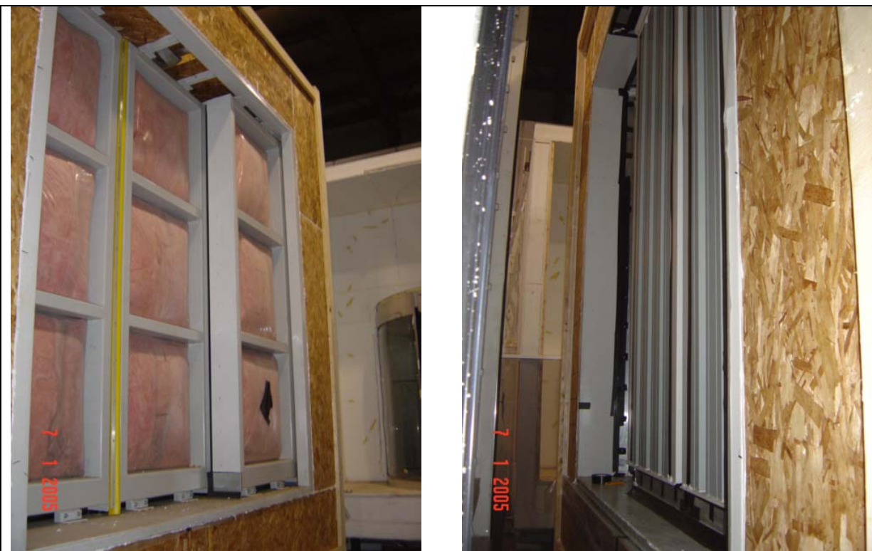
Figure 27 Specimen #7 installed in mask wall (viewed from interior and exterior)
