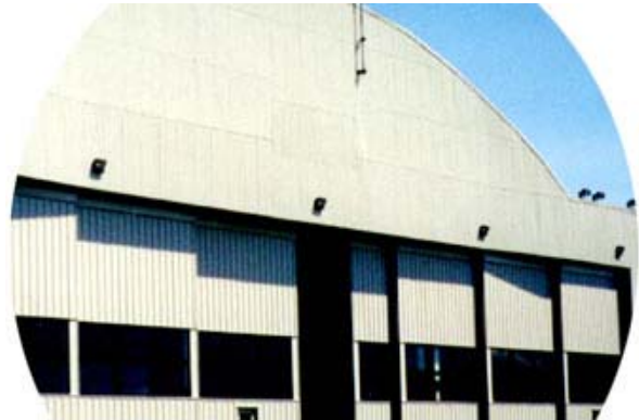
Figure 7 Typical aircraft hangar door
